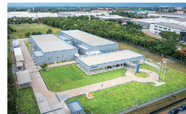
Mizuho(Thailand)Co.,Ltd. (Hi-Tech Industrial Estate, Ayutthaya)
